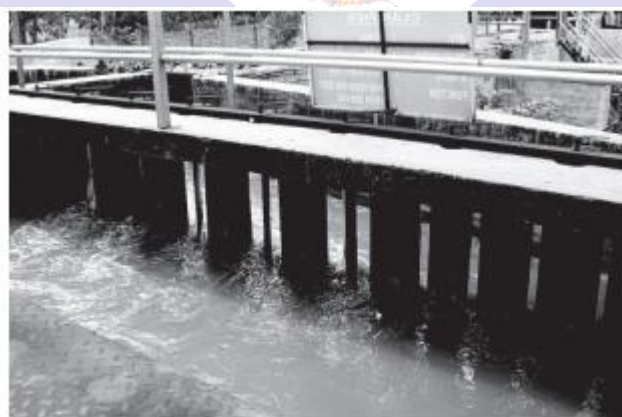
Fig. 18.4 Grit and sand removal tank
