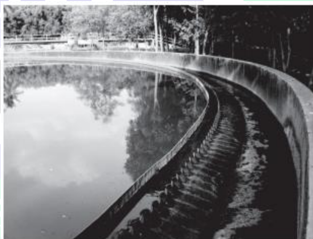
Fig. 18.5 Water clarifier
